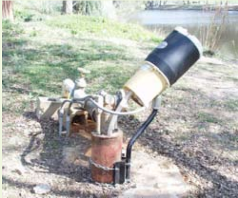
The LP-3000 dry pellet chlorinator is an easy way to chlorinate water for the purpose of controlling mussels. Chlorination also assists in decreasing sludge that forms inside pipes from precipitated iron and manganese.
